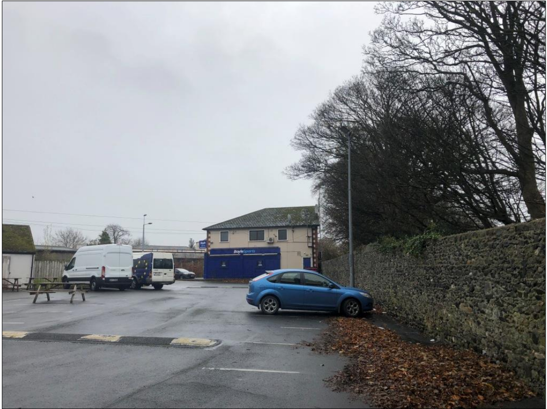
Image 6: Second view along the boundary wall showing the minor extent that which branches are overhanging the site.
