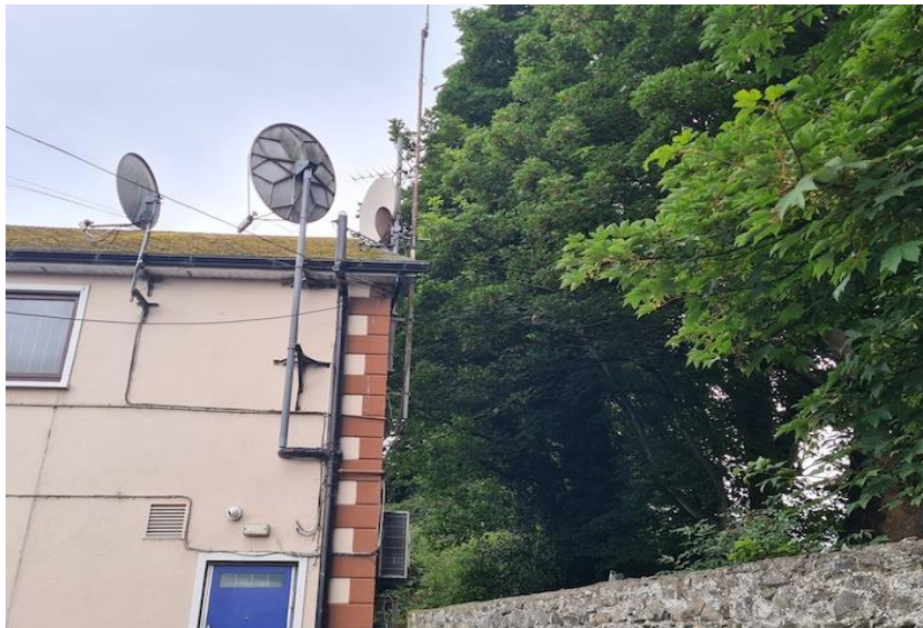
Fig. 2. Mature Sycamore Trees directly adjacent the buildings
