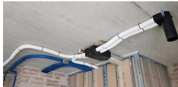
Figure 6 Typical apartment ducting system.
