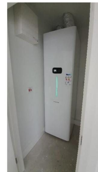
**Figure 1** Typical Exhaust Air Heat Pump (EAHP) Unit.
