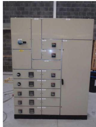
**Figure 8** Typical Form 4 main distribution board.
