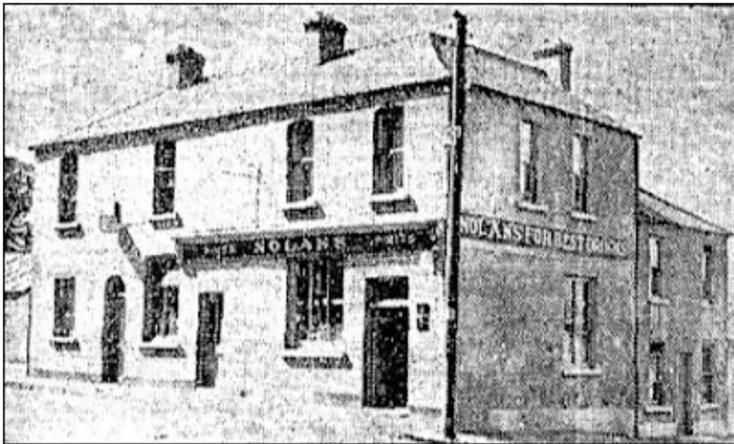
Plate No. 2. Historic photo showing Nolan's Bar, later known as the Firhouse Inn. At that time, the bar was only half as long along its primary elevation as it currently exists. A small single storey structure is barely visible to the left of the bar. Presumably this was the Smithy, or Forge, later to be demolished when the two-storey structure was extended to the west.
