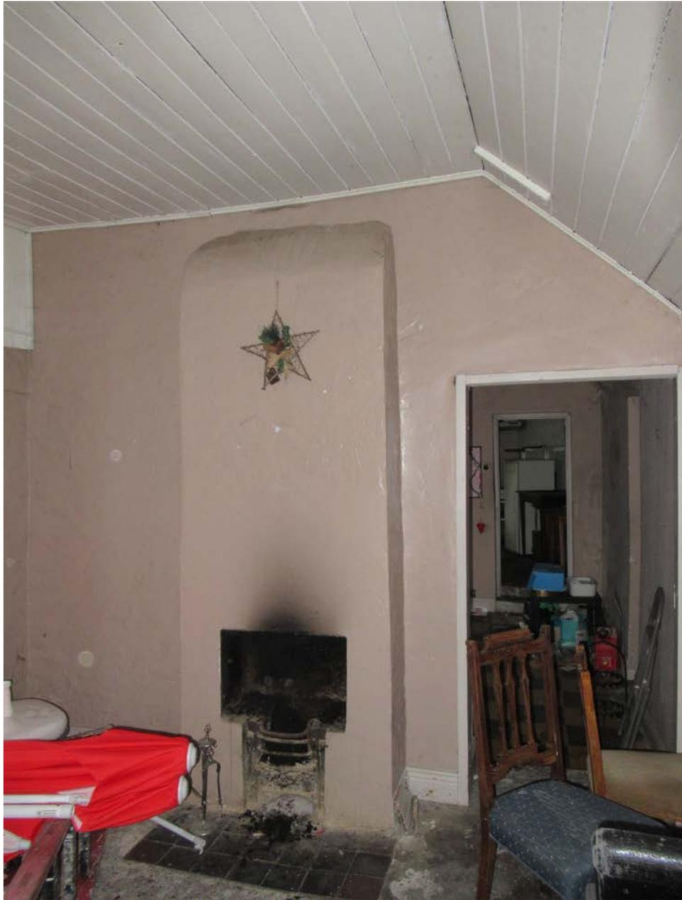
*Plate No. 11. General internal view showing the chimney breast in the east room in the cottage. Note the timber-sheeted ceiling, with the collar ties raised above the wall heads.*
